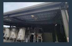
The netting that was installed did not have the edges sealed and made the situation worse.
